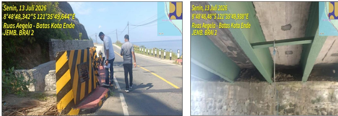
Figure 1. Field survey documentation of Brai 2 Bridge, 13 July 2026: (a) bridge and safety barrier viewed from the roadway; (b) composite steel girders viewed from beneath the structure, coated with protective paint in May 2026 as a preventive measure to reduce further corrosion.
